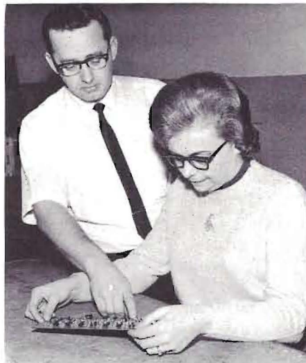
NEW PRODUCT —Thelma Stewart, assembler in Department 979, and Calvin Yeaton, Senior Engineer, Department 143, look over the complex wiring of a Timing Generator Circuit Pack for the D2 Channel Bank, a new product which is soon to go into production at the Merrimack Valley Works.
