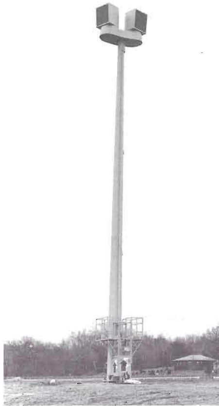
A cable car on the side of the new BTL installation near the athletic field provides easy access to experimental equipment.
