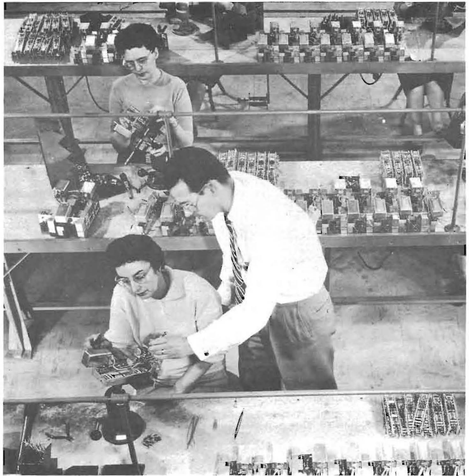
Wiring operation of "317" components used in "O" type carrier terminal equipment.
