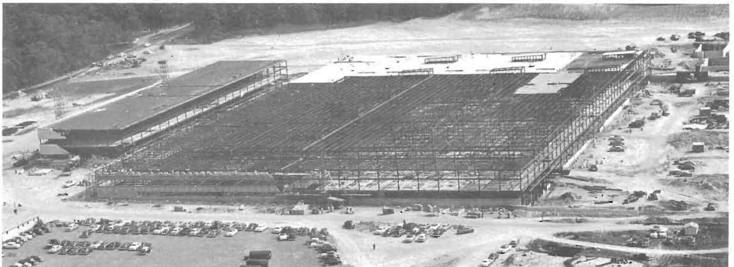
Initial construction of the Merrimack Valley Works in 1956.
