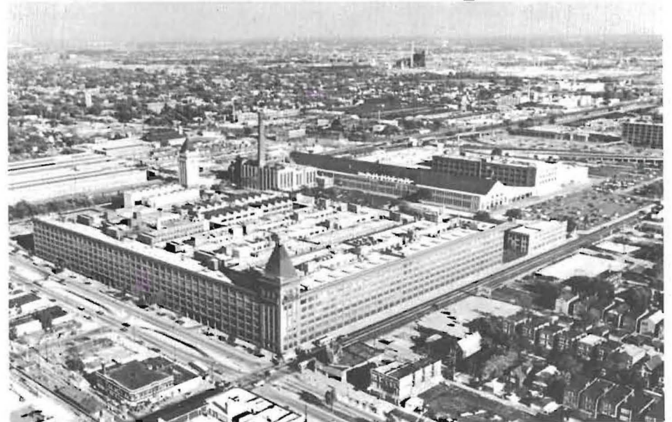
HAWTHORNE WORKS in Cicero, Ill., is pictured here on its 163-acre site, where a large shopping mall is planned. The location's famed tower, lower center, has been a landmark for many years.
