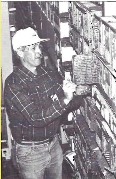
Bob Nolan, engineering planning and development DACS technical customer support manager, examines fire damaged packs.
